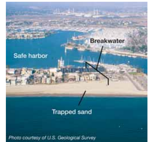
Figure 12.9: A breakwater is a barrier to longshore drift that protects harbors. Excess sand can build up near a breakwater.
